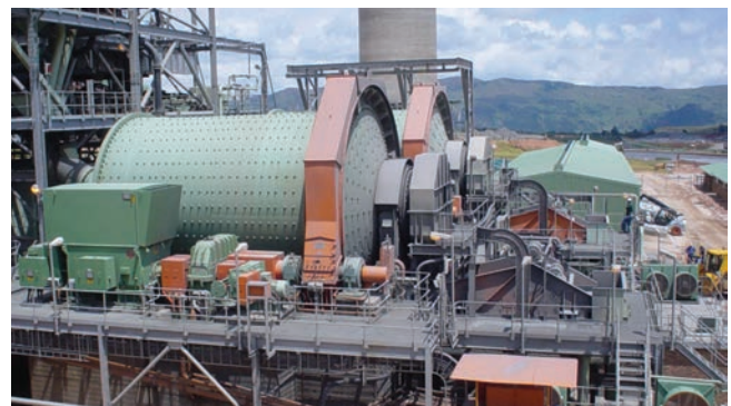
Everest South Platinum Mine Single Pinion Mills: WRIM with Brush lifting device + Liquid Rheostat Starter
